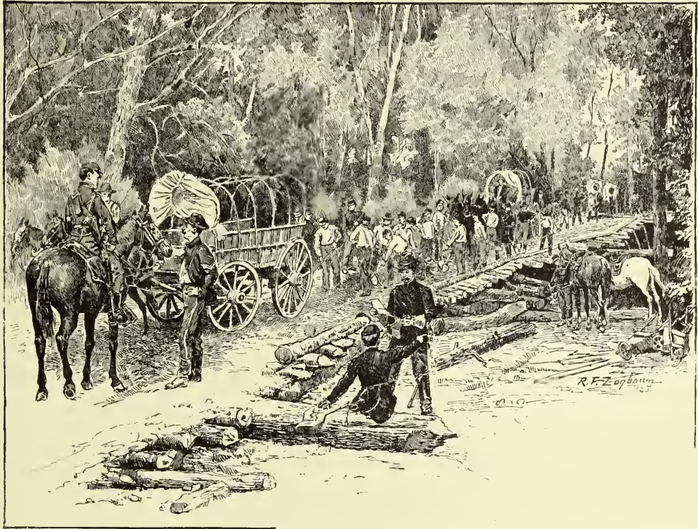
UNION TROOPS BUILDING THE CORDUROY APPROACHES TO GRAPEVINE BRIDGE. FROM A WAR-TIME PHOTOGRAPH.
